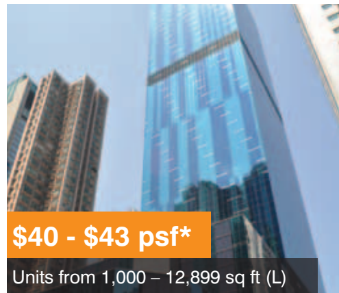
AIA Tower 183 Electric Road
